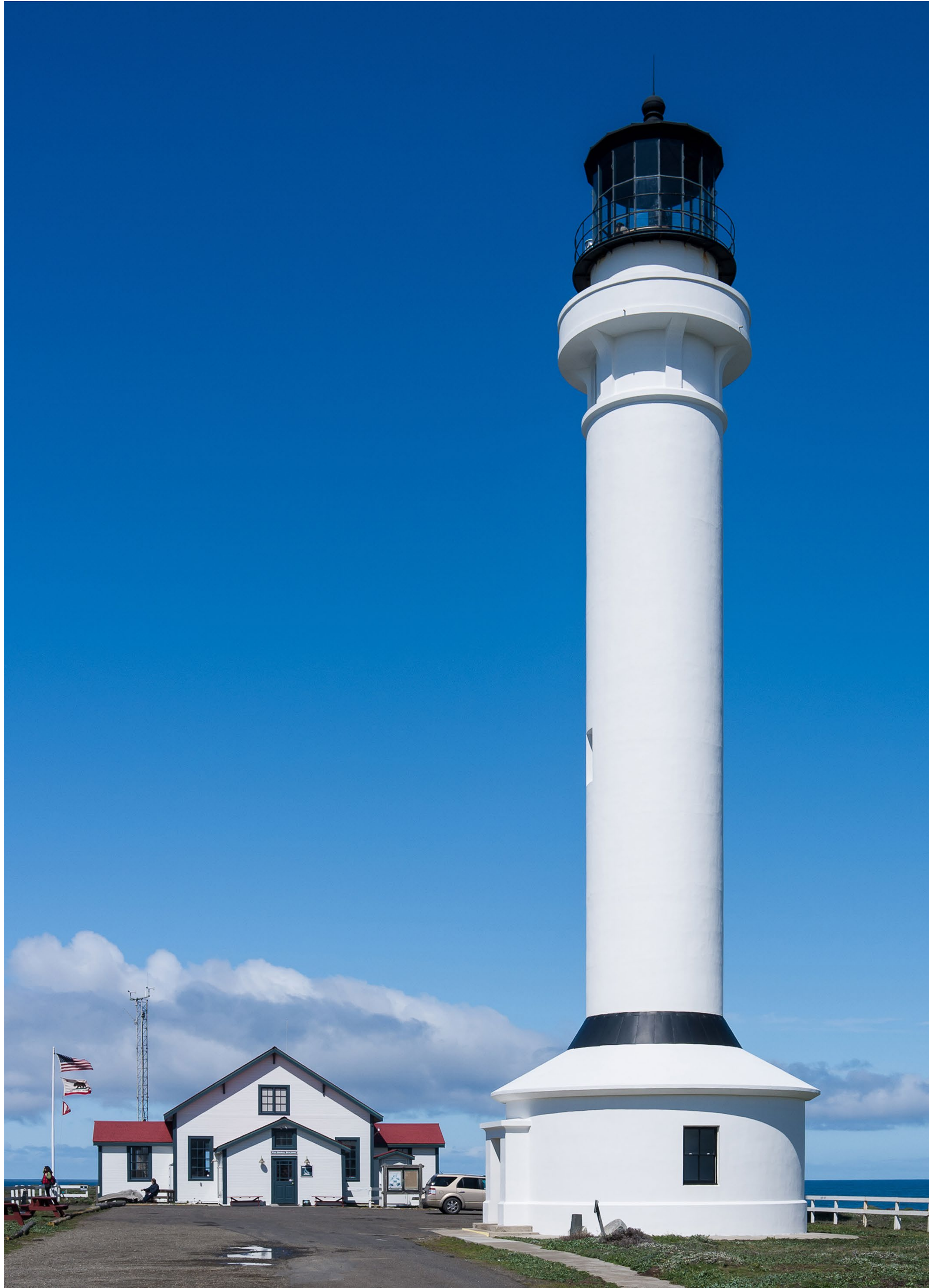
POINT ARENA LIGHTHOUSE AND FOG SIGNAL BUILDING
